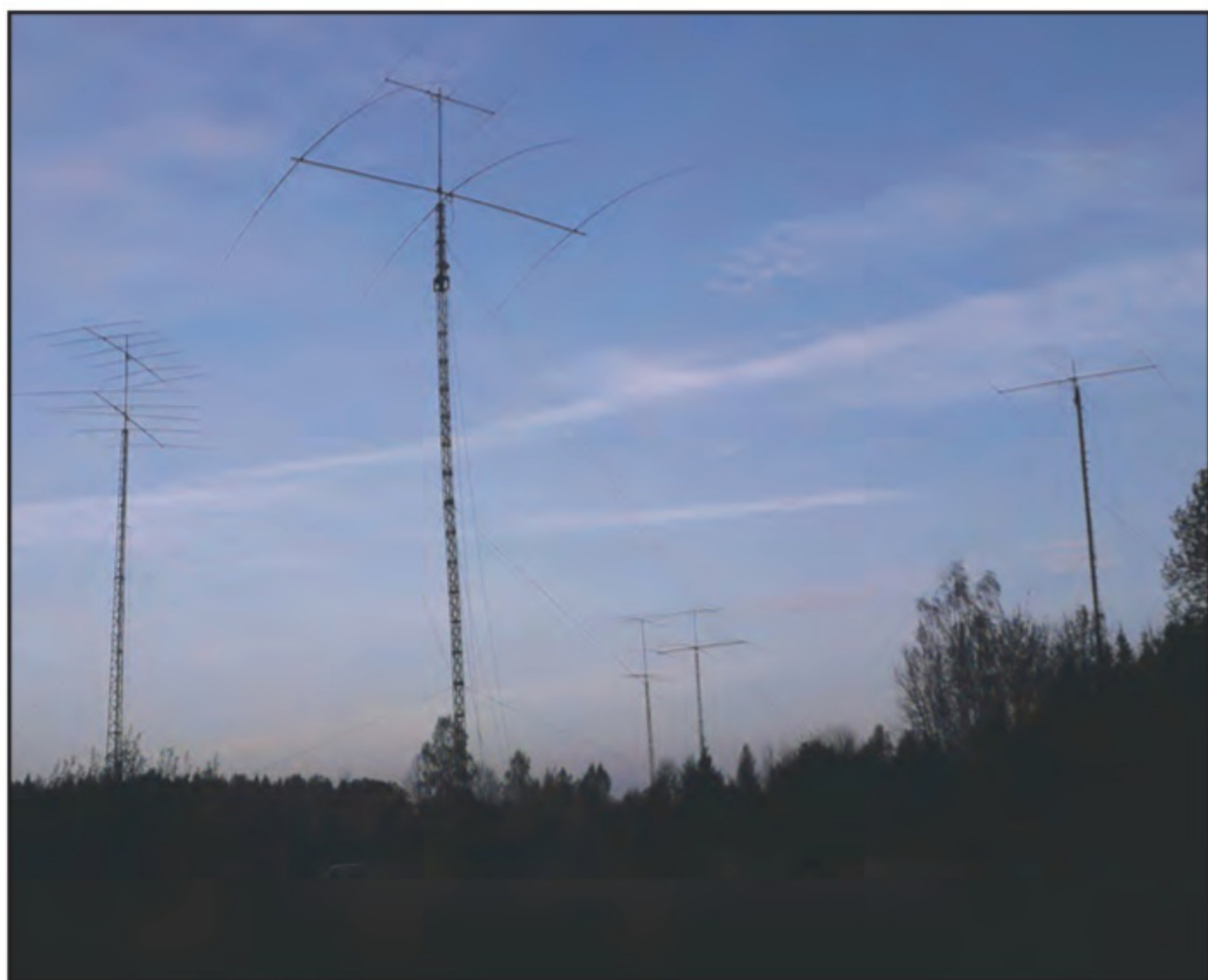
LY9Y's antenna farm.
